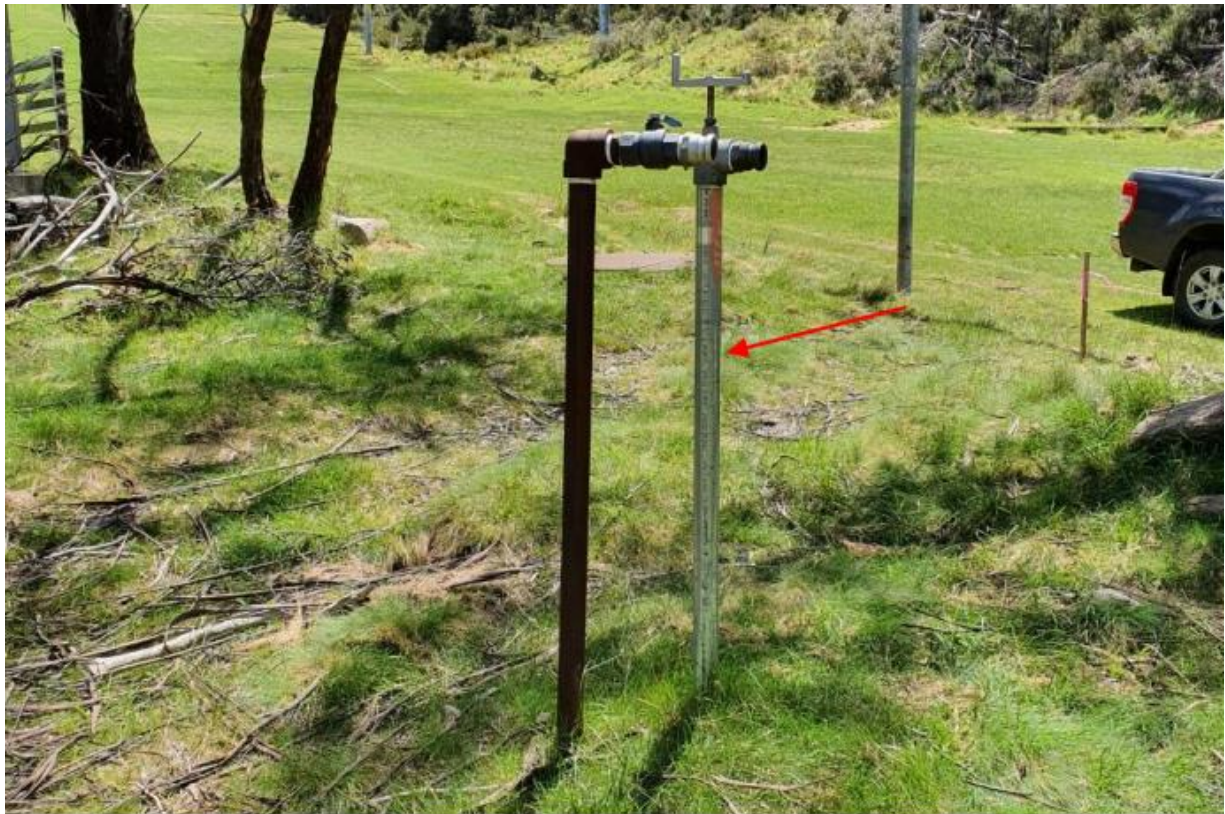
Figure 8 | Example of manual hydrant installation (Source: Applicant's documentation)
