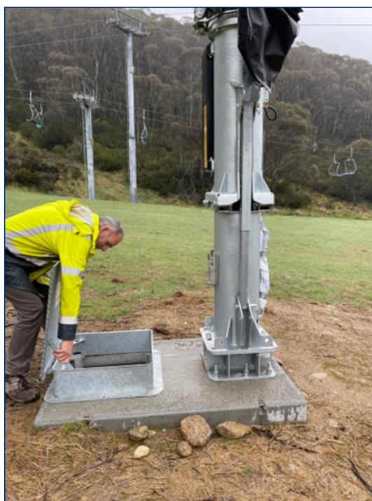
Figure 10 | Example of snowmaking gun installation on concrete pit (Source: Applicant's documentation)
